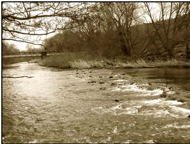
Figure 3c: Buck Mill and weir site and footbridge, 2006
