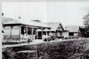
A general view of the Open Air School
